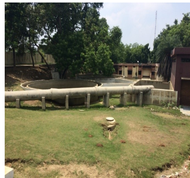
Figure 23: Balaganj Back Wash
