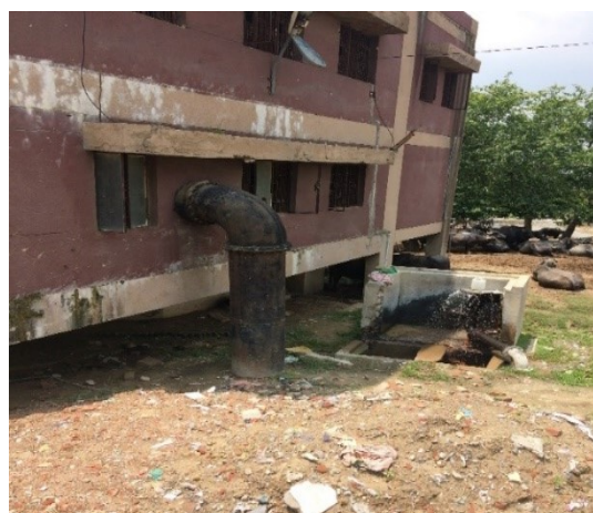
Figure 74: Pipeline snapshot field survey
