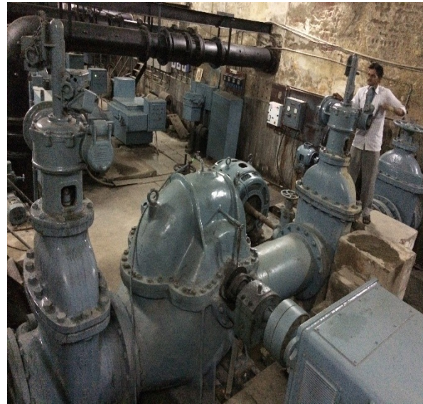
Figure 10: Pumping Station 2 (for 650mm & 500mm dia. pipe line)
