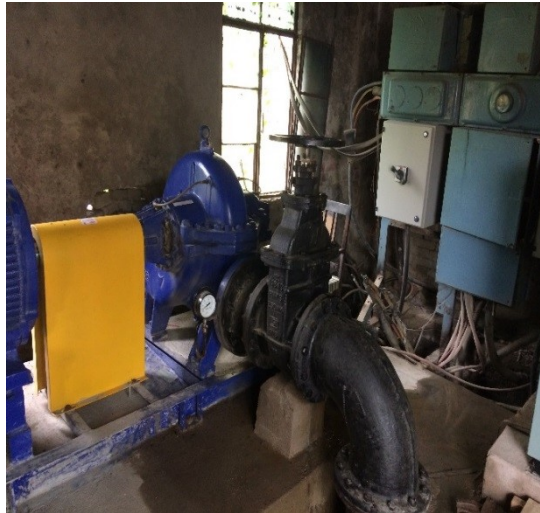
Figure 19: Aishbagh Pumping Station 4
