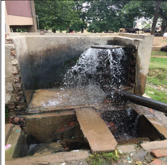
Figure 38: Leakages of Balaganj WTP
