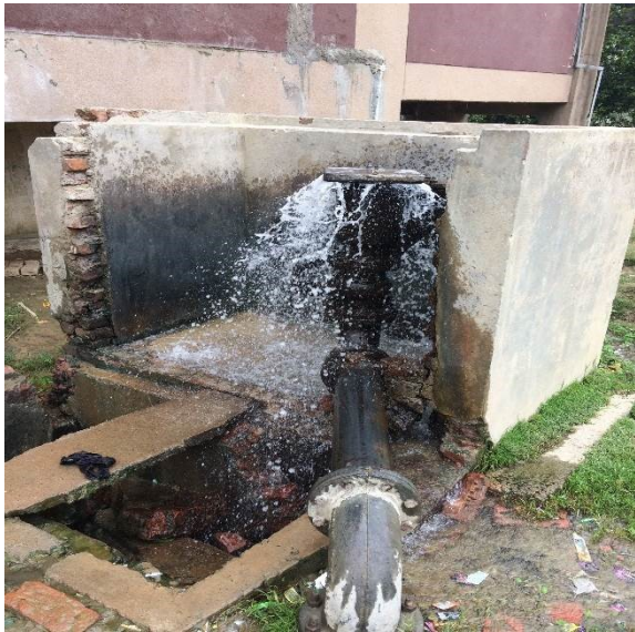
Figure 76: Leakage in air valve at Balaganj WTP
