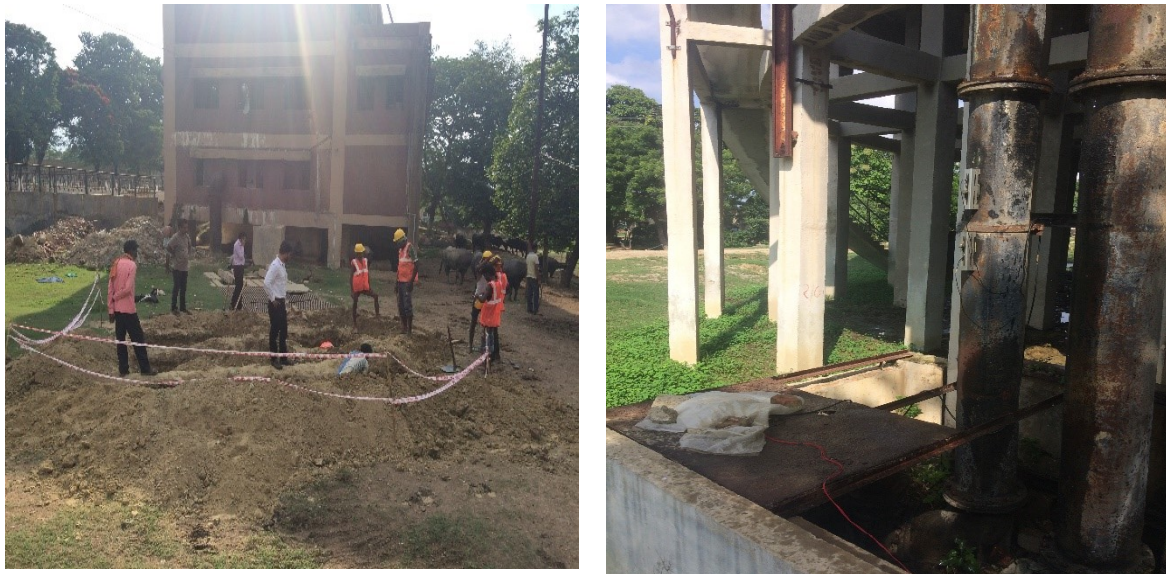
Figure 37: Balaganj WTP Flow Measurement
