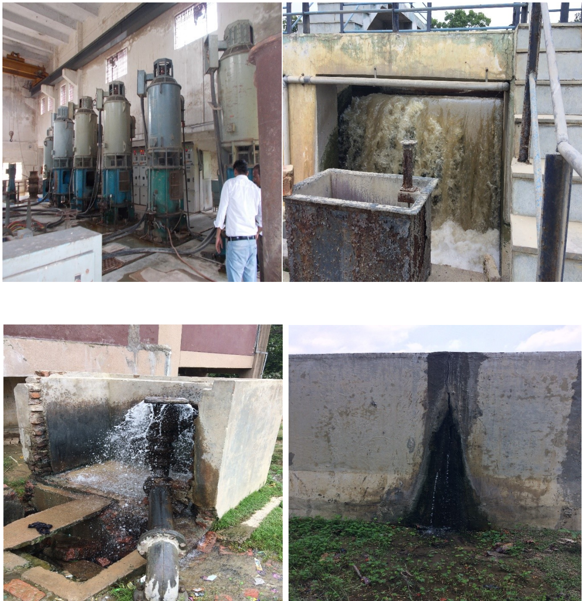
Figure 27: Leakage in settling tank
