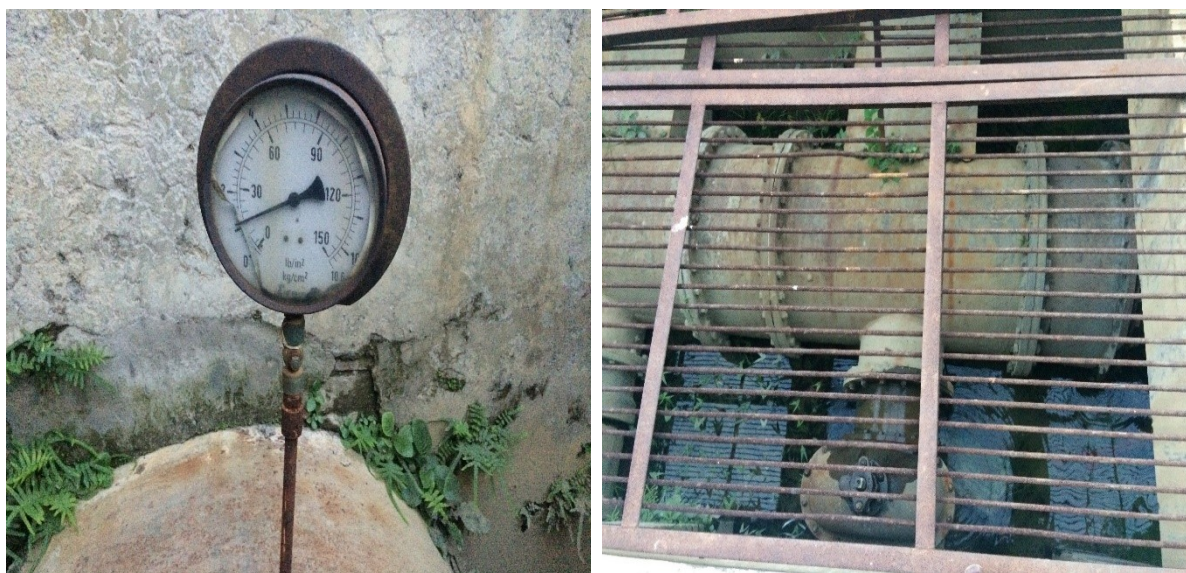
Figure 17:Aishbagh Pumping Station 2
