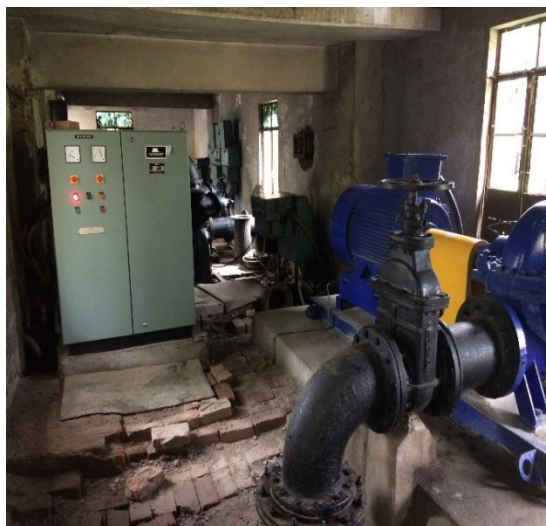
Figure 18: Aishbagh Pumping Station 3
