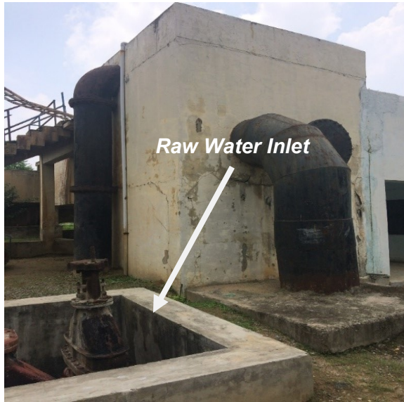
Figure 21: DN 900 Raw Water Inlet at Balaganj
