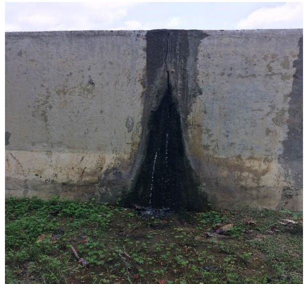
Figure 77: Leakage in settling tank at Balaganj WTP
