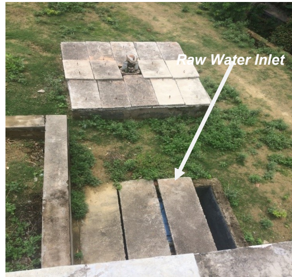
Figure 20: DN 1200 Raw Water Inlet at Balaganj
