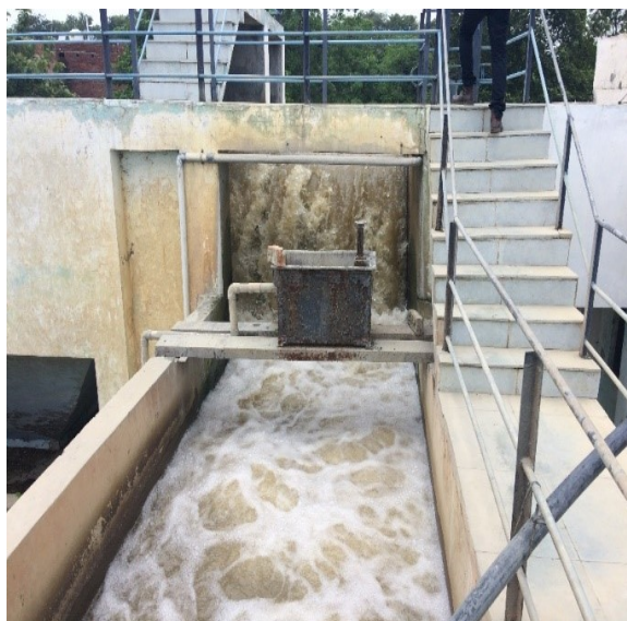
Figure 22: Water Inlet in Water Works
