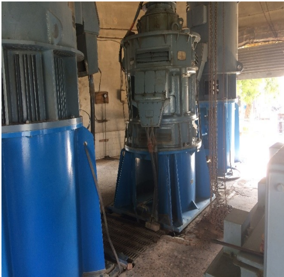
Figure 11: Pumping Station 1 (for 1300mm & 1200mm dia. pipe line)
