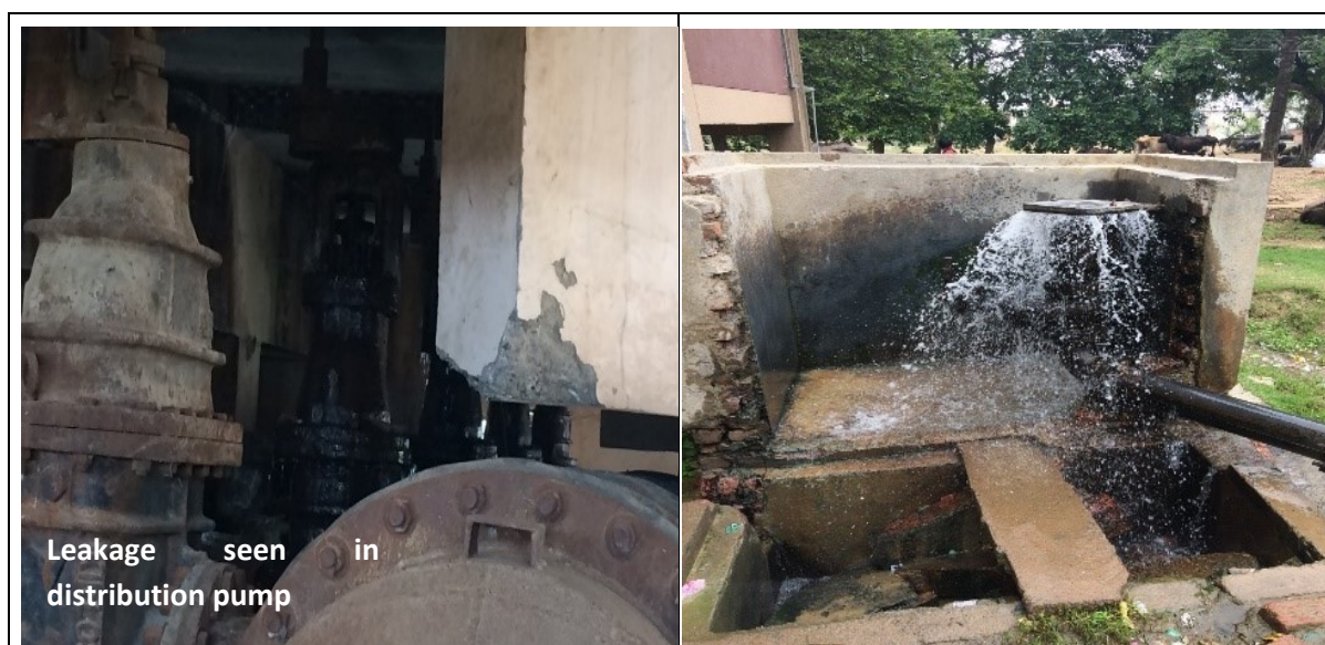
Figure 28: Leakage in Air valve at the outlet
