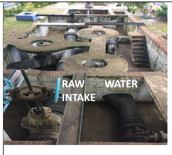
Figure 15 Raw Water Supplied from Gaughat Pumping Station
